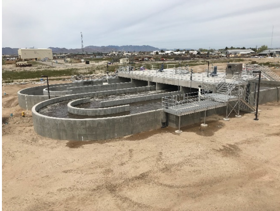
Newly constructed oxidation ditches at the Willcox WWTP
