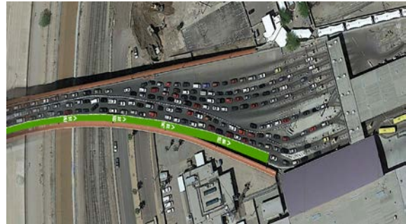
Analysis of a proposal for better infrastructure and operations – Development of Executive Project.
