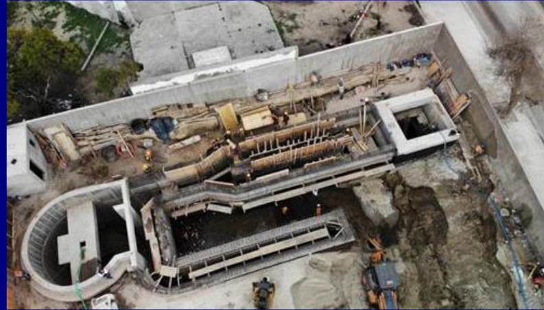
New grit and trash removal pretreatment
