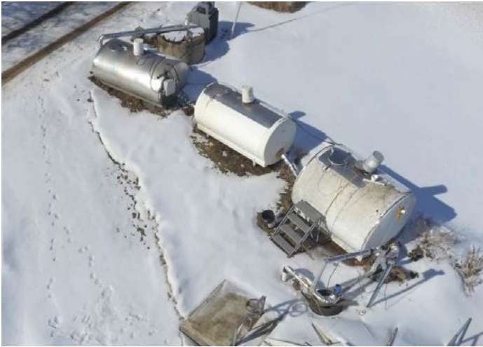
Blenker-Sherry POTW's Milk Tank Pre-Anoxic Zone
