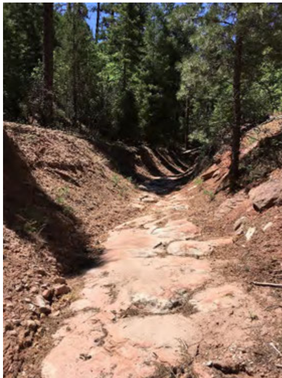
Figure J5-46. DC3A: View of the drainage near SD12
