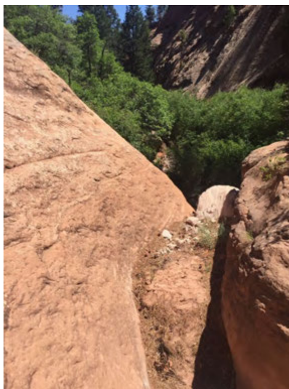
Figure J5-6. DC1: View of drainage at SD23.
