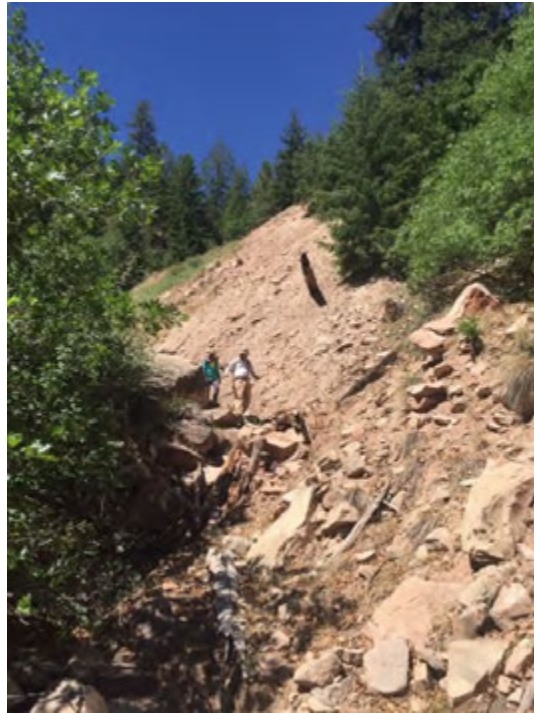
Figure J5-20. DC2B: View of the waste pile above Middle 2B drainage.
