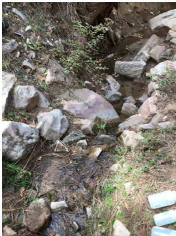
Figure J5-61. DC3E: Drainage at DC3E near SD10
