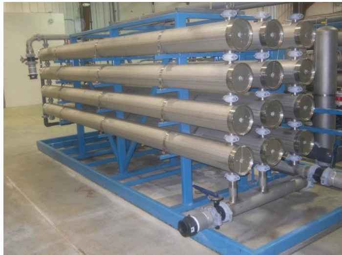
A skid of reverse osmosis filters
