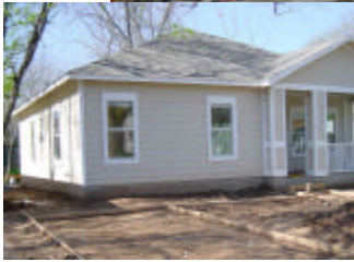
SMART Projects in Austin, Texas. Photo provided by City of Austin.
