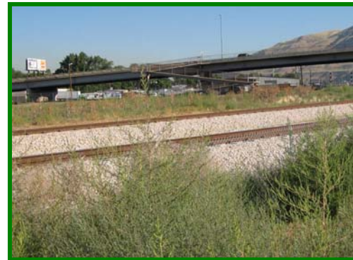
View north from the middle of the Parcel. The North Temple viaduct is visible in the background, and the new Frontrunner Commuter Rail tracks are visible in the foreground. The Union Pacific freight train tracks have been moved west (to the left).
