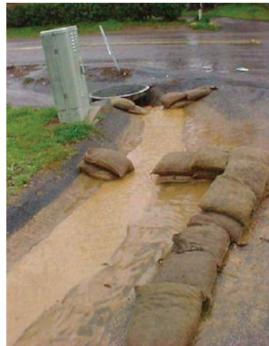
Figure 5. Make sure storm drain inlets are protected.
