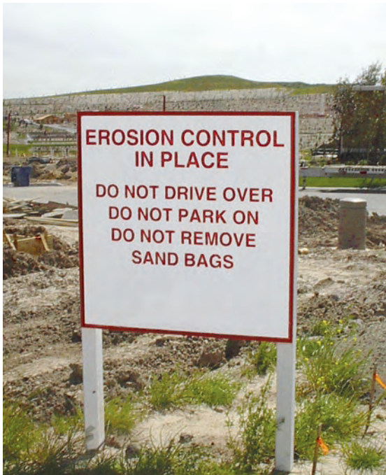
Figure 4. Use signage to help educate construction staff.
