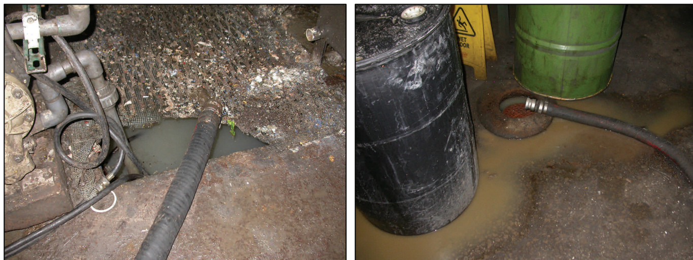
Hose used to discharge hazardous waste into illicit tank and drain.
