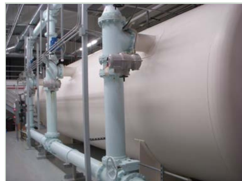
High Pressure Filtration, Flint Lake Drinking Water Plant
