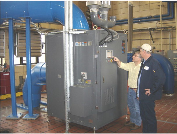
Facility staff monitor the energy gains of new high-efficiency turbo blower.
