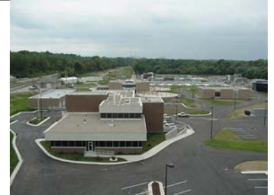
Lafayette Wastewater Treatment Plant
