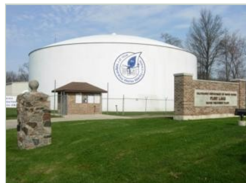
Storage, Flint Lake Drinking Water Plant
