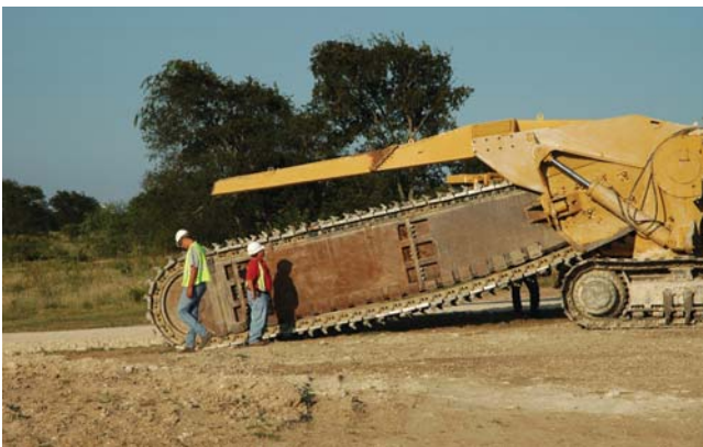
Trenching Machine Used in Biowall Construction
