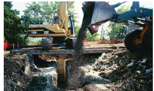
Media Backfilling of Biowall Trench
