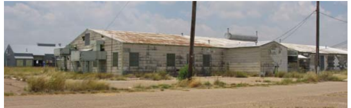
Formerly Used Military Building
