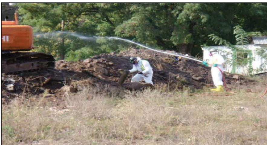
Superfund contractor wetting suspected asbestos containing material from the dump site.
