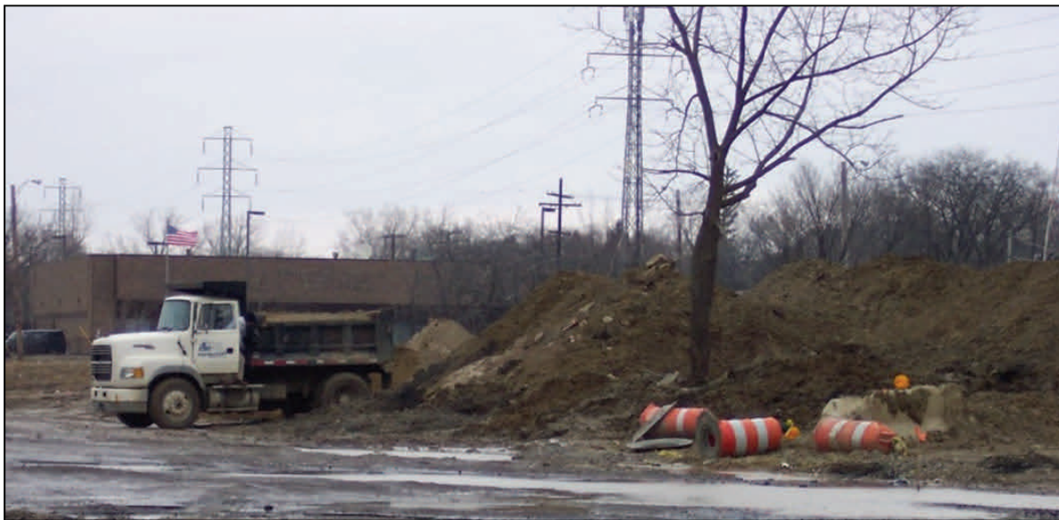
Mountains of soil brought to the HUD site.
