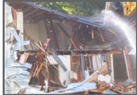
As an outcome of the field testing, the CCLRC staff was able to illustrate the need for additional field oversight. Two additional staff members joined the CCLRC team to focus on contractor performance in the field.
