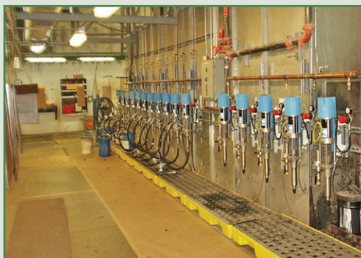
Stain Booth, After the Project
