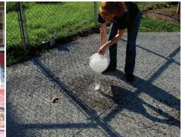
Figure 68 porous concrete sidewalk
