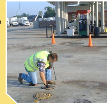
Inspecting a spill bucket
