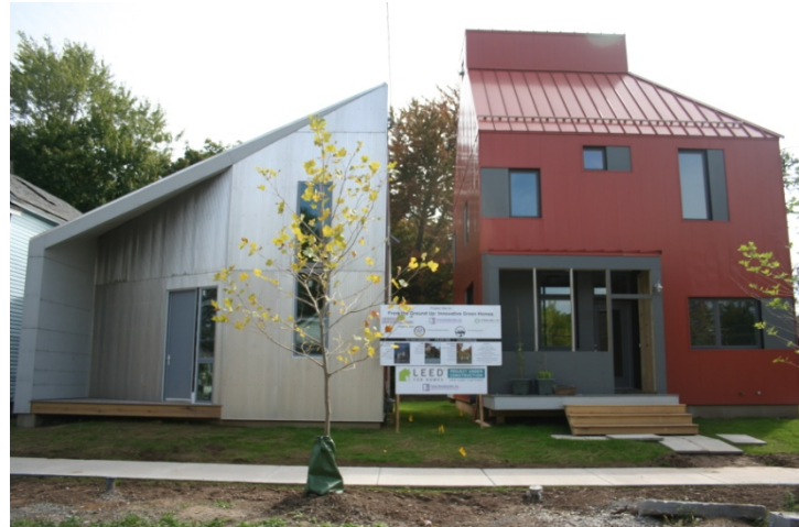
Figure 4. Single-family homes under construction in Syracuse, New York. These homes were built within an existing residential neighborhood not far from the city center. Photo credit: Syracuse Center of Excellence.
