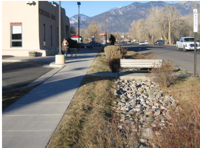
Figure 16: The planted buffer makes the sidewalk feel safer and more comfortable for pedestrians.
