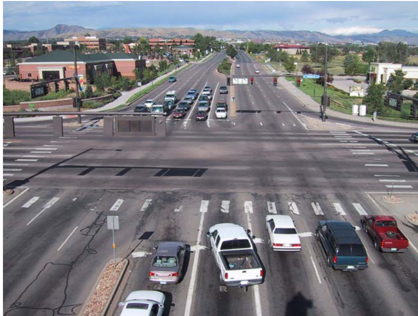
Figure 19: An example of a suburban-style street. The version suggested for this section of the Paseo would have fewer lanes than shown here: two travel lanes in each direction and one left-turn lane at major intersections.
