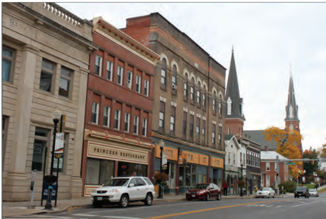
Figure 11: Frostburg's Main Street is next to residential neighborhoods and Frostburg State University. The new SRF selection criteria helped the city get funding for a project that will encourage growth nearby, putting new homes within walking distance of jobs, stores, and restaurants.
