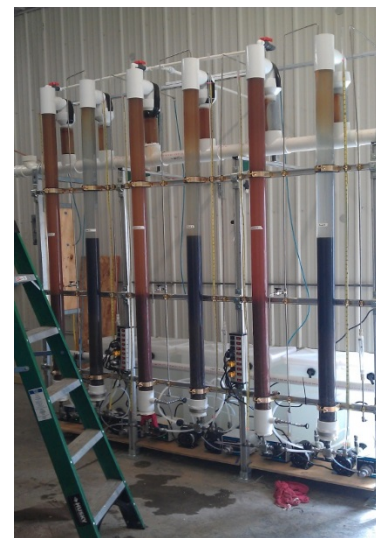
Figure 3. Pilot biological water treatment system for ammonia removal at the Palo, Iowa study site.
