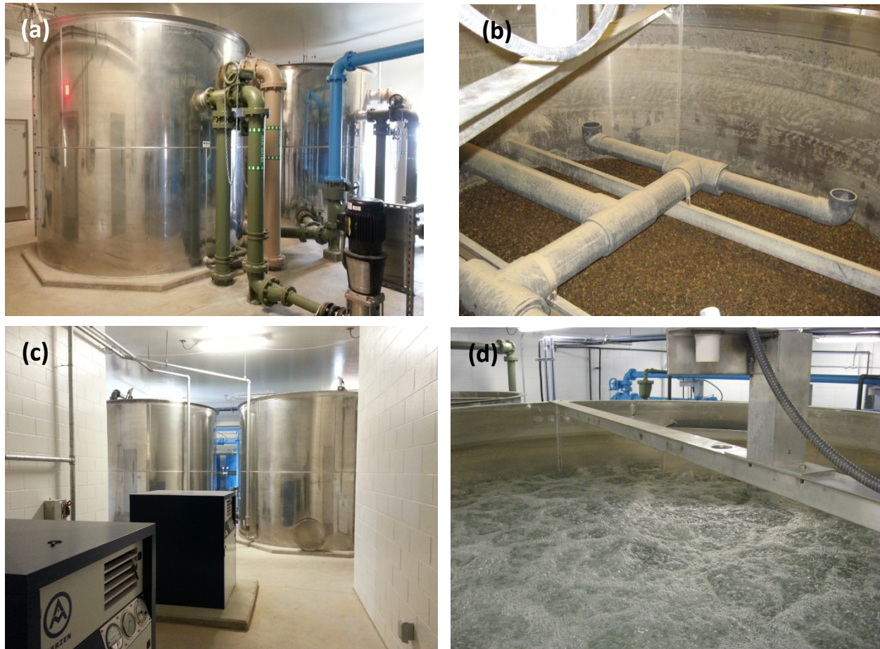
Figure 6. Photographs of (a) aeration contactors, (b) contactor media and piping, (c) aeration contactors and air blowers, and (d) aerated contactor surface.
