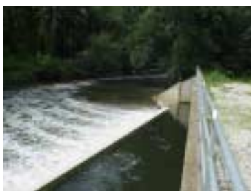
Left – Akron WPCS discharge to Cuyahoga River.
