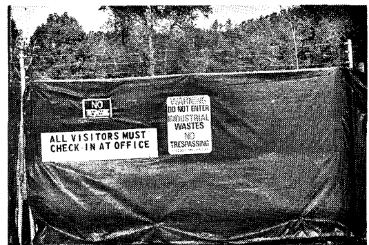
The Michigan Avenue dump site clean-up
