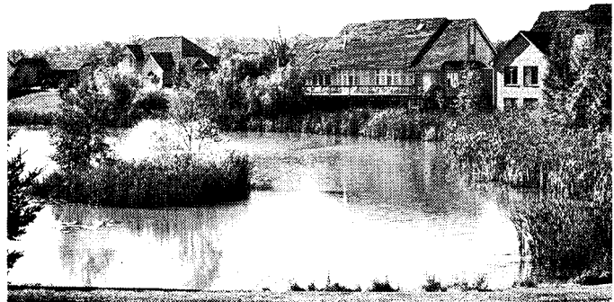
Stormwater retention basin, W. Bloomfield
