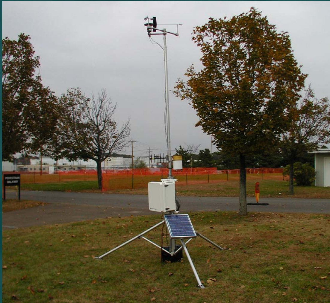
Example of Tripod Weather Station
