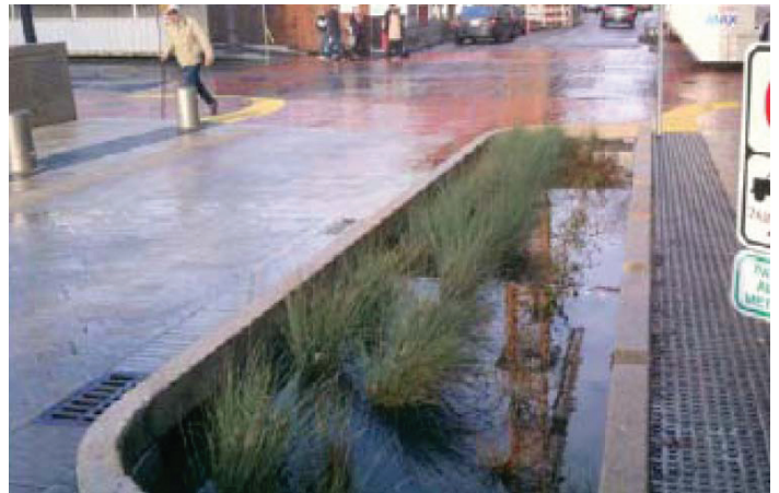
Right of way detention basin. Source: U.S. EPA Office of Brownfields and Land Revitalization
