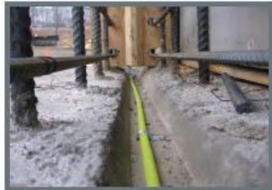
Figure 5. Anchoring clips on injecto.
