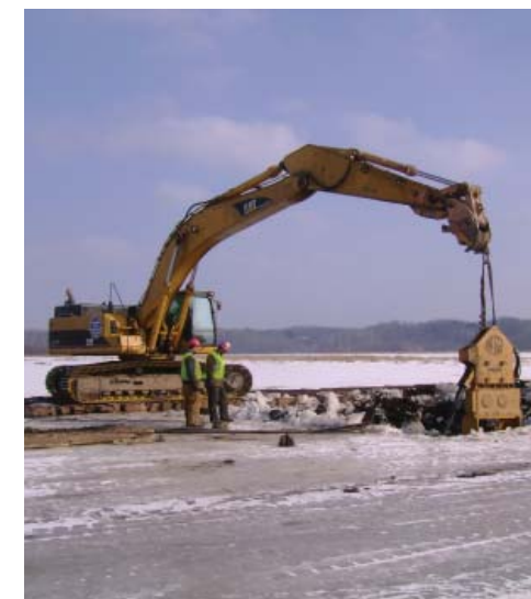
Removing pilings in Radio Tower Bay. Photo by SLRA
