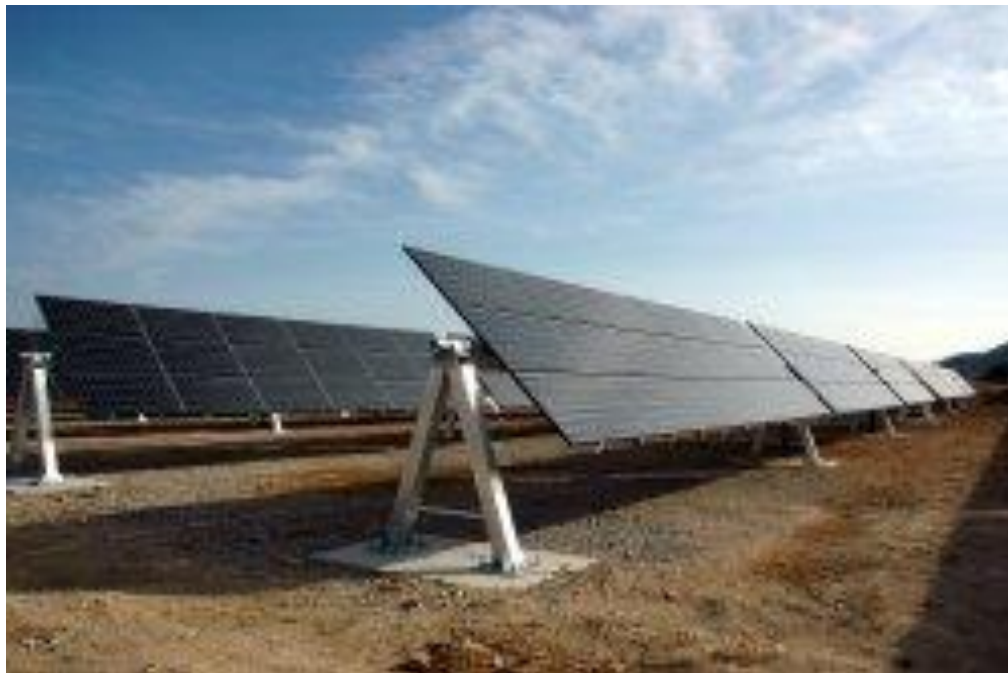
Figure 3. Example of Single Axis Tracking Mount
