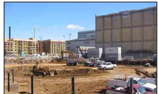
Soil excavation underway at the Fox Courts property.
