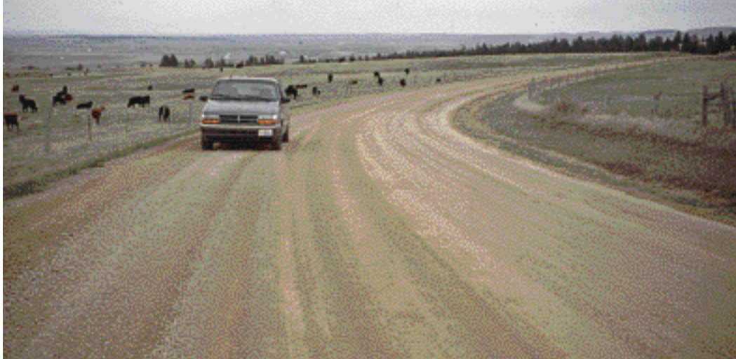
This superelevated road section makes driving safer.
