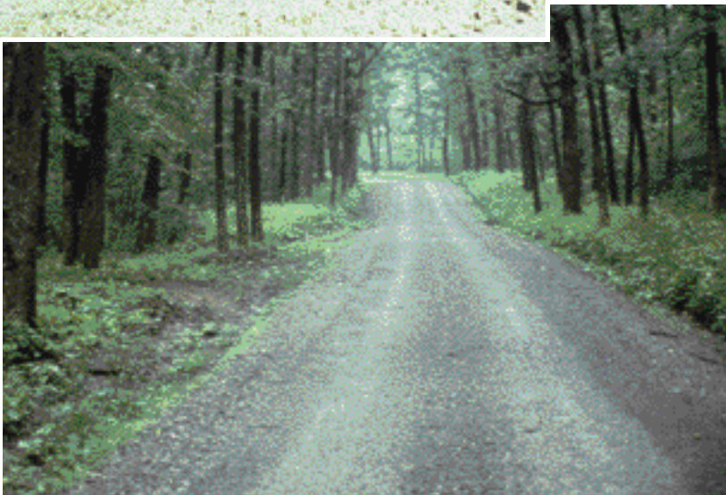
The road now performs very well after the stabilization was completed.
