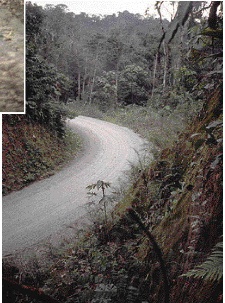
This well-traveled road in Ecuador performs well in a region that receives approximately 200 inches average annual rainfall. (Courtesy of Ron Anderson, Tensar Earth Technologies, Inc., USA)
