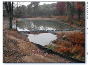
Figure 1. One of a series of limestone treatment ponds installed.
