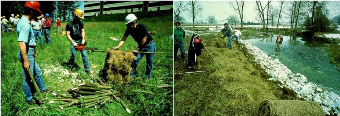
6.35 Cutting the stakes and Preparing the site.
