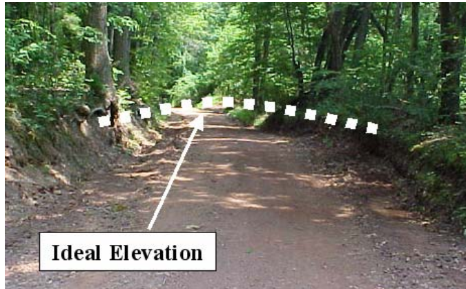
ESMP12-01 A typical entrenched road.
