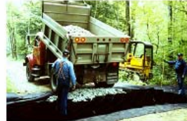
↑ Dumping aggregate fill ↑
