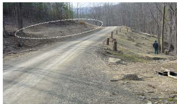
6-31 Newly constructed low-gradient bank benches.
