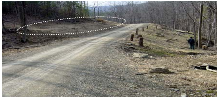
ESMP#13-04 Newly constructed low-gradient bank bench.
