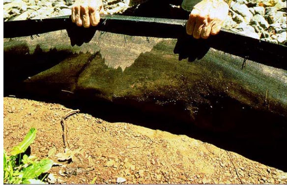
ESMP#15-01 Separation fabrics keep the soil and road aggregate in place.
