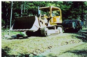
↑ Compacting the aggregate ↑
