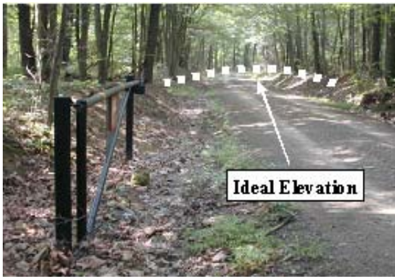
Before, an entrenched road
