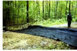
↑ Placing fabric ↑
