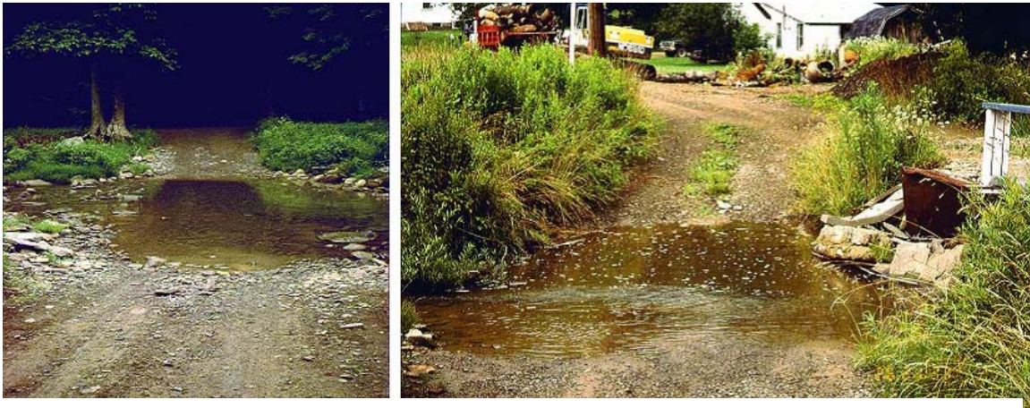
5-33 Existing fords should be stabilized to prevent erosion and stream degradation.
