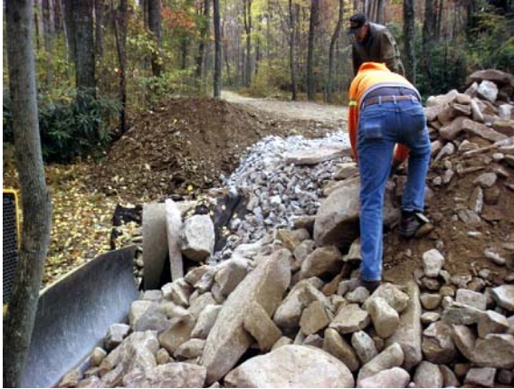
A7-08 Placing large size riprap at ends of pipe.
