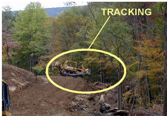
ESMP#13-03 Tracking newly constructed banks.
