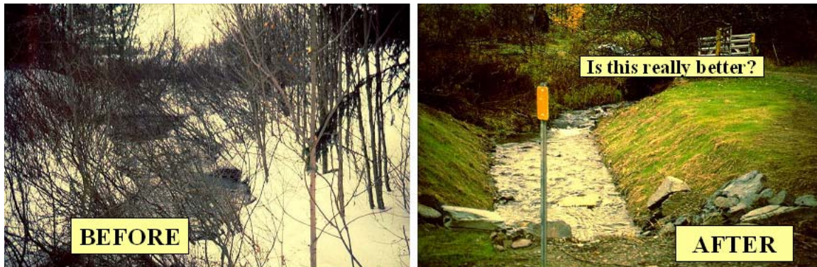
6-17 Clearing stream banks for a road crosspipe replacement can have devastating effects on the stream and future maintenance.
