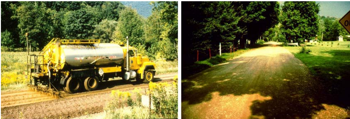
7-10 Road stabilization or full-depth reclamation works well with a stabilizing agent
