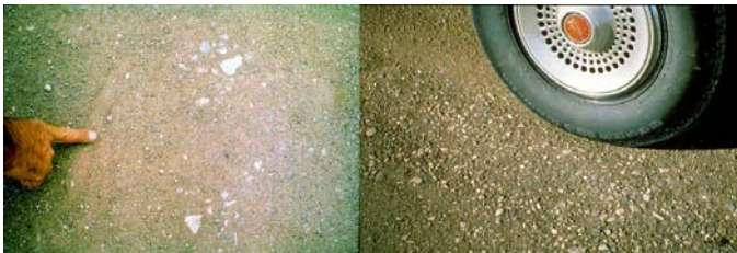
3-18 Good road surfaces differ in appearance depending on aggregate type and gradation.
