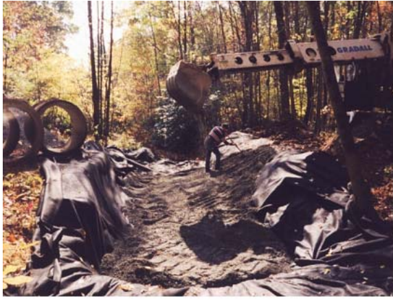
A7-04 Bedding material added
