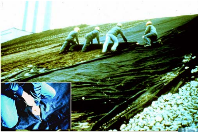
7-24 Installation of an erosion control fabric.
