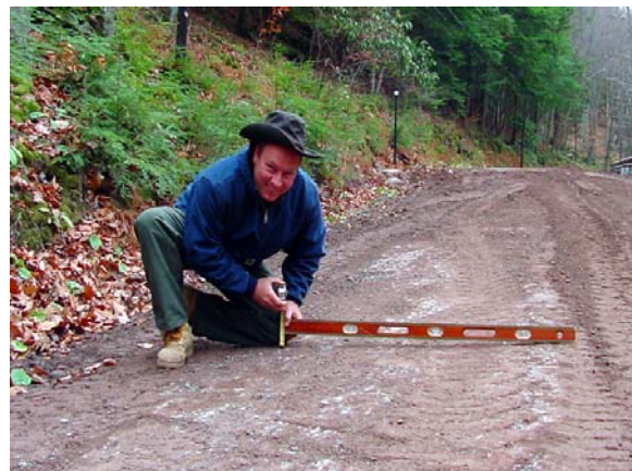
3-20 Checking Cross Slope to insure proper drainage.
