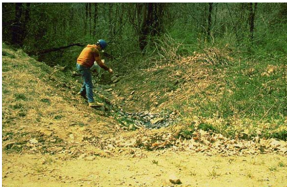
5-13 Seeding and mulching may be sufficient to revegetate the ditch.
