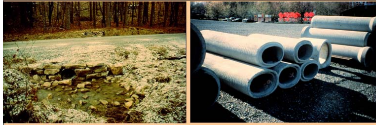
Figure 1: For shallow installations, use rigid pipe, pipe arch, or elliptical concrete (rigid) pipe
