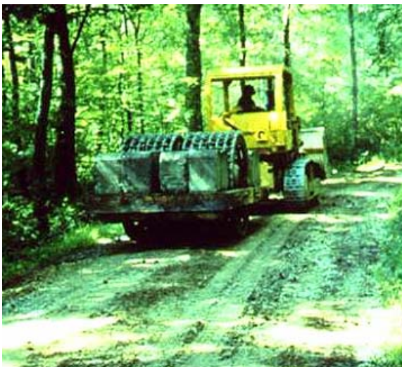
7-15a A steel grid-type roller fractures large coarse shale material.
