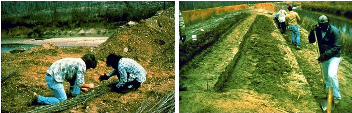
6.38 Tying the bundles and digging the trench.
