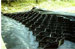
↑ Geocell ready for fill ↑
