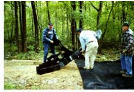
↑ Placing geocell ↑
