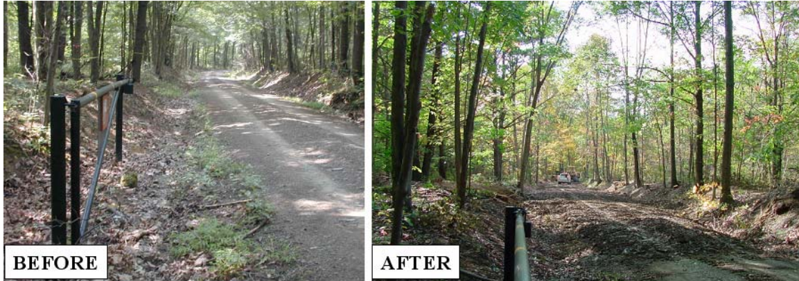
ESMP#14-05 A before and after look at selective tree trimming during a road project – using the forest system to reduce maintenance.
