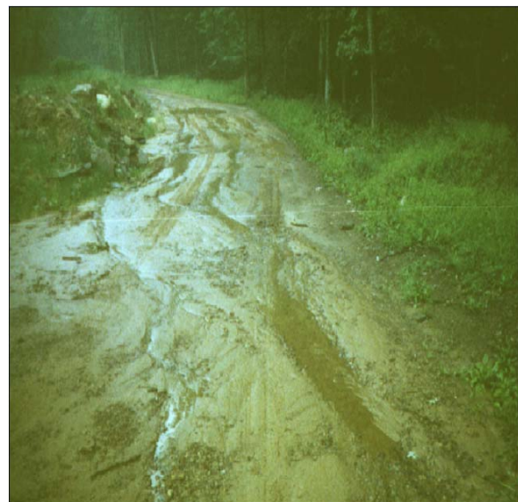
3-06 Spring, “Mud Season,” can be a trying time for road maintenance crews.
