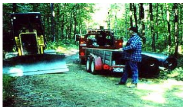
↑ Rolls of fabric waiting for installation ↑
