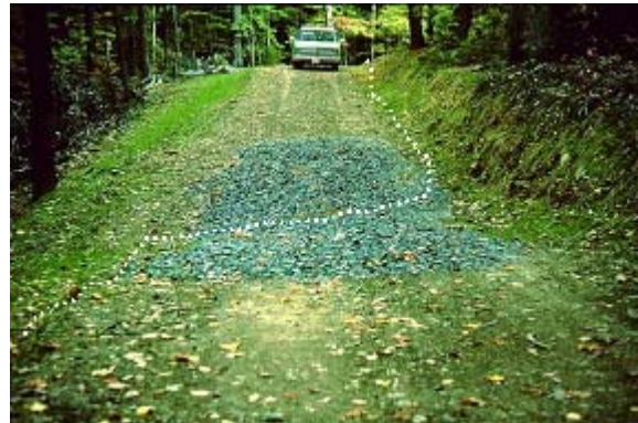
5-23 Broad based dip reinforced with large aggregate.
