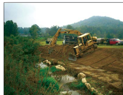
Figure 2. Implementing a stream restoration project on a Clear Creek tributary.
