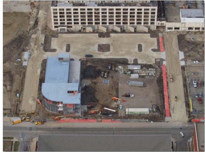
Construction of Creative Technology Accelerator Building Courtesy CityWide Development
