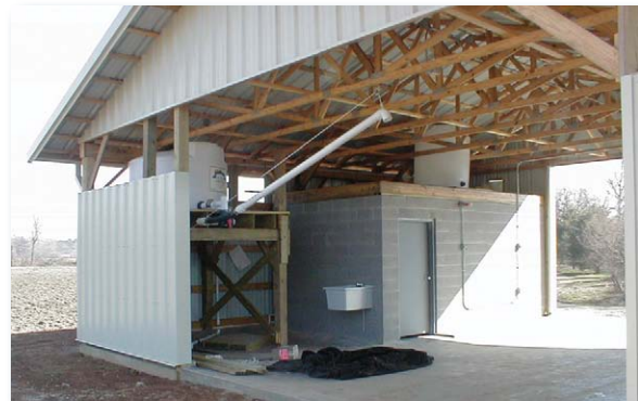
This chemical-handling facility replaced one that was directly adjacent to Mills River.
