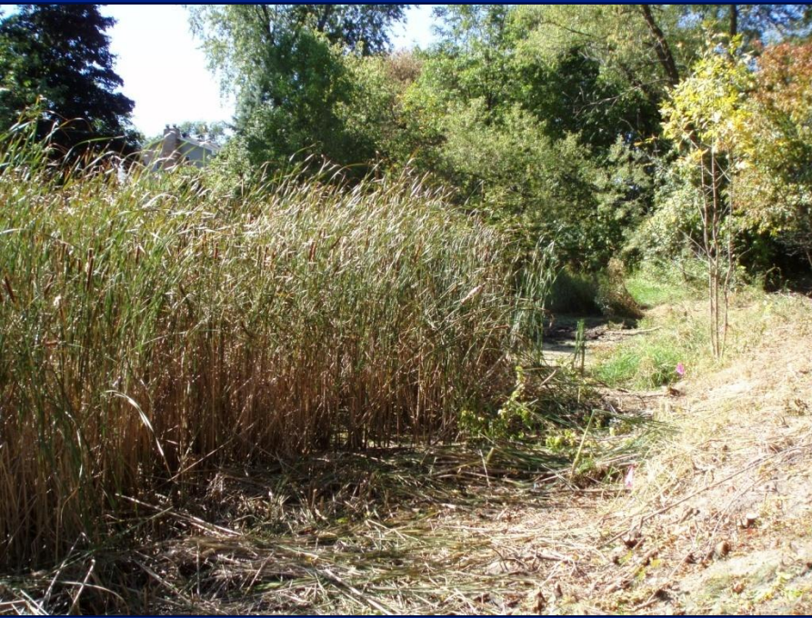
Nonfunctioning stormwater ponds in Woodbury, MN
