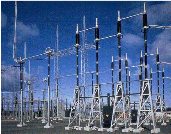
Figure 1: 735 kV AIS
