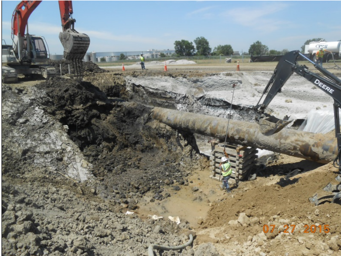
Photo 1: Technica excavating impacted material south of the pipeline near Area ARA-W.
