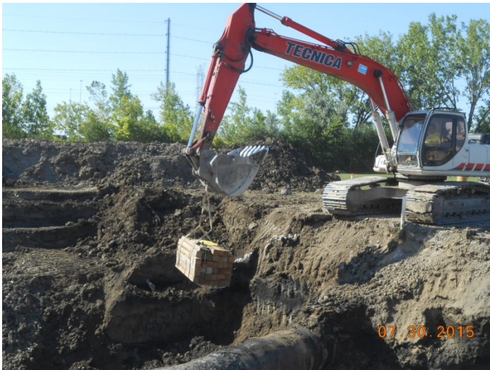
Photo 2: Installation preparation for the pipeline support cribbing.
