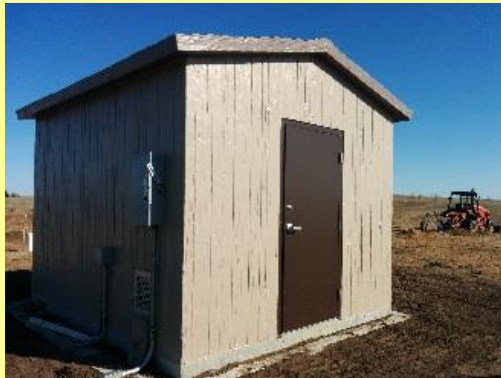
New well house in Beverly. (EPA OIG photo)
