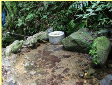
Portillo Miramar water system's surface water intake. (EPA OIG photo)
