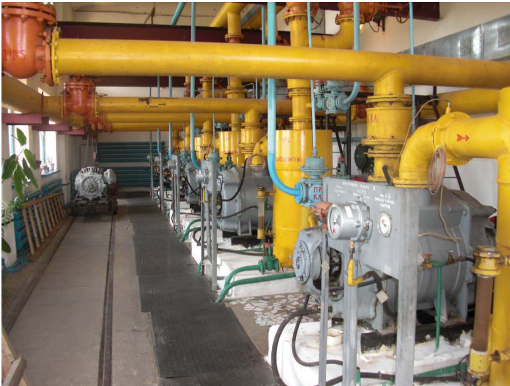
Figure 5. LRVP extraction station
