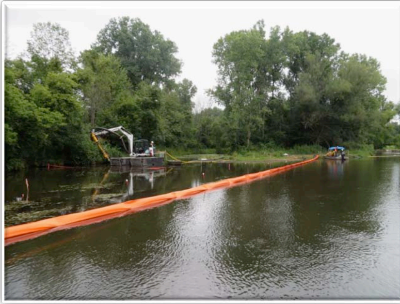
Figure 73 – Sediment Removal via Vacuum at MP 10.40 (8/2/2013)
