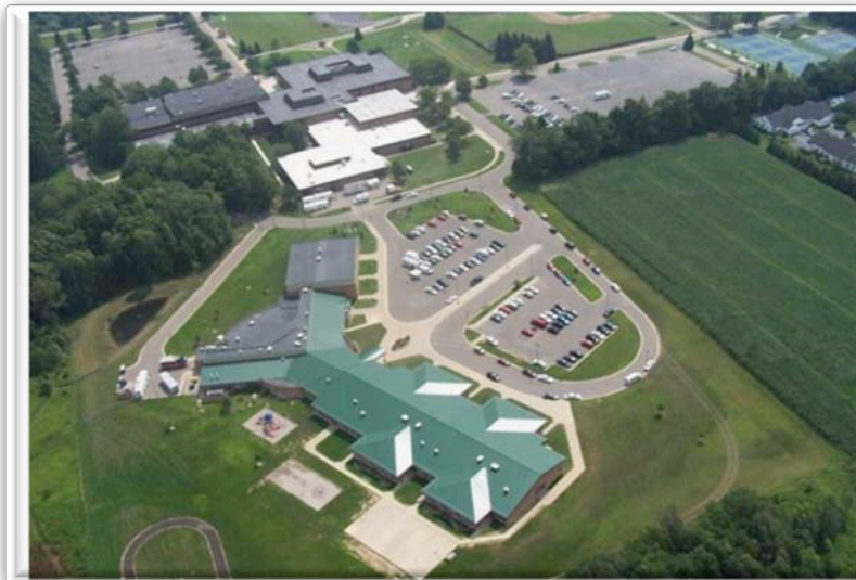
Figure 101 – Walters Elementary School ICP
