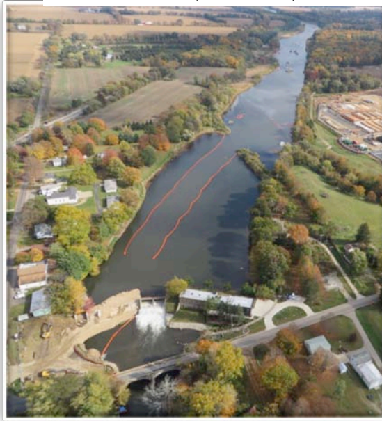
Figure 35 – Ceresco Impoundment Dredge Area Prior to Notching Ceresco Dam (10/18/2013)
