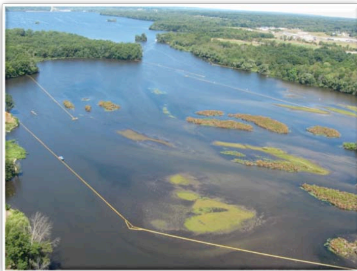
Figure 59 – E4 Containment Structure at Morrow Lake Neck (7/10/2012)
