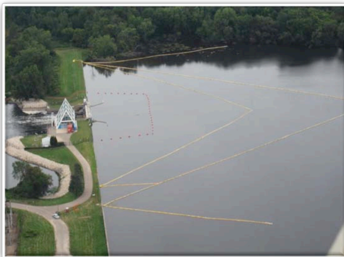
Figure 17 – Double Chevron Boom Upstream of Morrow Lake Dam (8/14/2010)
