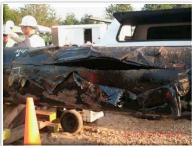
Figure 2 – Ruptured Portion of Line 6B Pipeline
