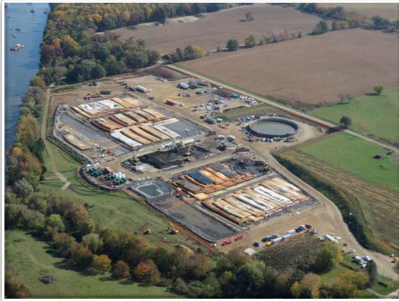
Figure 34 – Sediment Dewatering and Processing Pad at Ceresco Impoundment (10/18/2013)
