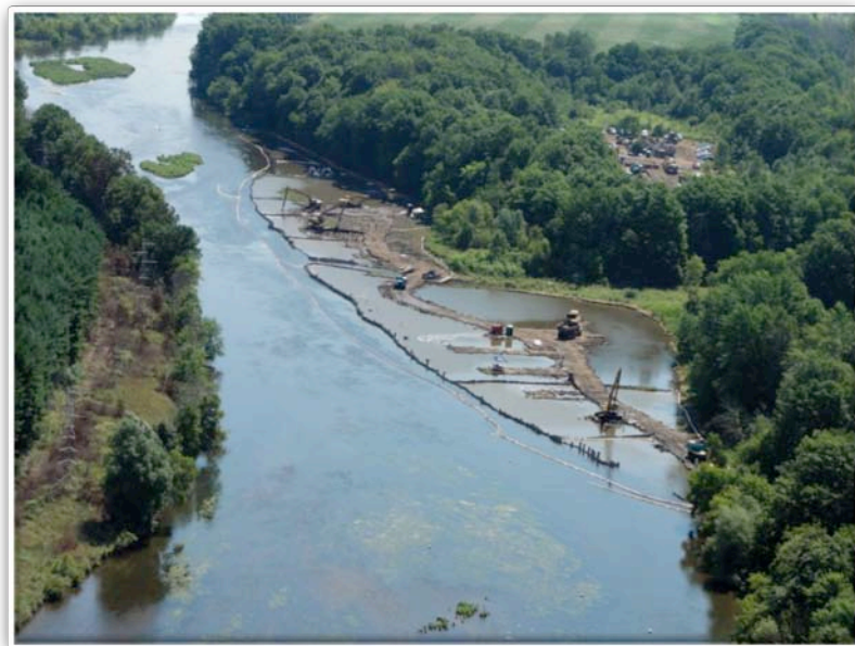
Figure 47 – Excavation of MP 4.50 LDB (8/9/2011)
