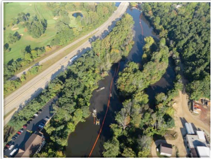
Figure 38 – Dredge Unit Operating at the Mill Ponds Impoundment (9/25/2014)
