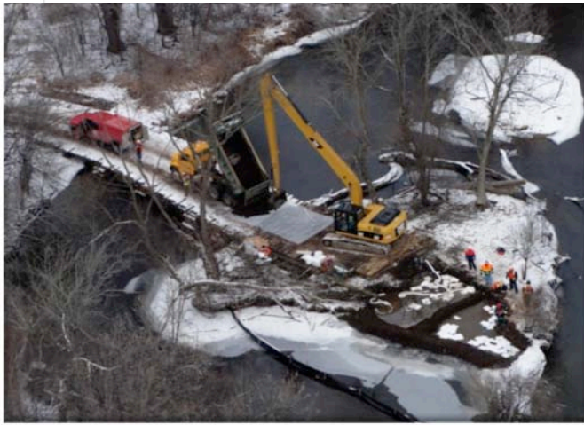
Figure 44 – Excavation of MP 2.75 Island during Winter 2010 Overbank Recovery Activities
