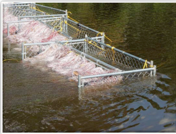
Figure 18 – Gabion Basket in the Kalamazoo River (1/28/2012)
