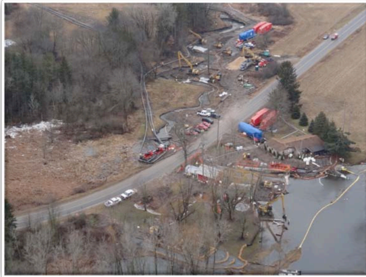
Figure 51 – Excavation of Talmadge Creek at the Confluence with the Kalamazoo River (3/1/2012)
