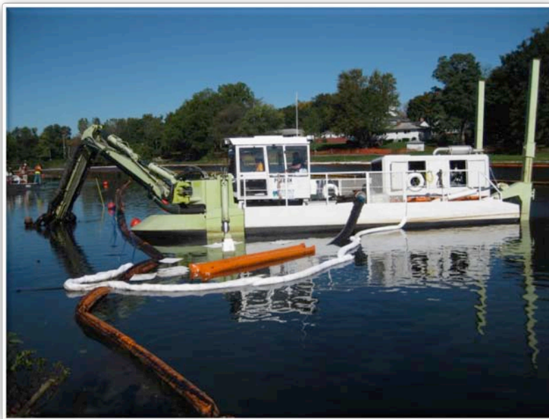
Figure 22 –Dredging at MP 5.75 Ceresco Impoundment (9/30/2010)
