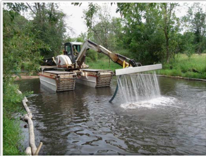
Figure 28 – Excavator with Hydraulic Spray Bar Agitating Sediment (7/28/2011)
