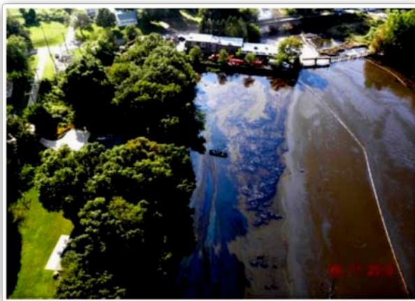
Figure 1 – Discharged Oil Accumulating Upstream of Ceresco Dam (7/26/2010)
