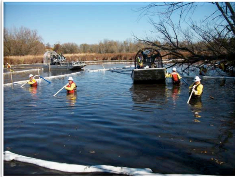
Figure 21 – Oil Recovery via Sediment Agitation using River Water (10/16/2010)
