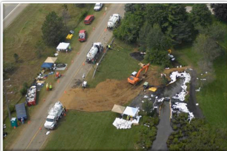
Figure 13 – Recovery Actions and Devices at Talmadge Creek (8/2/2010)
