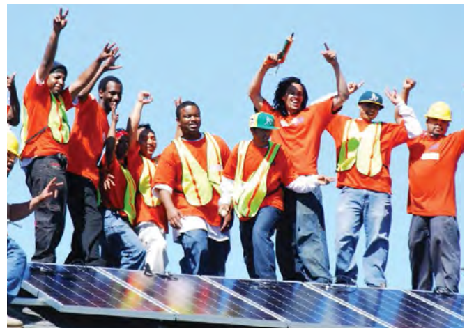
RichmondBUILD participants complete a solar installation project.
