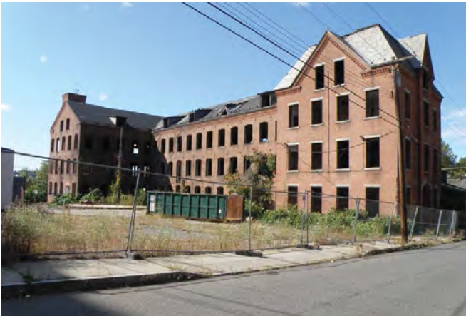
More than 80 percent of the non-hazardous building materials were recycled during a deconstruction project at the Cherry Street Industrial Park in Waterbury.
