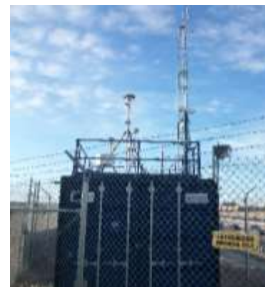
Air monitoring station tower along the I-15 highway corridor in Las Vegas, Nevada. (EPA photo)
