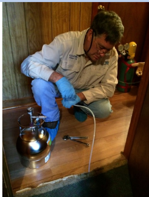
Right: Sub-slab sampling inside a home in May 2016
