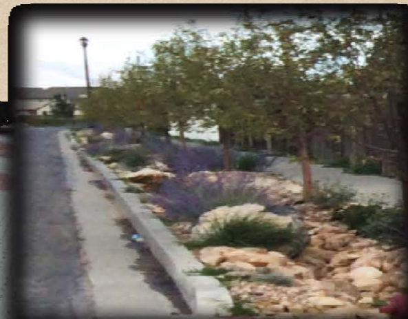
Shallow Infiltration w/out Pretreatment (D- blocks)
