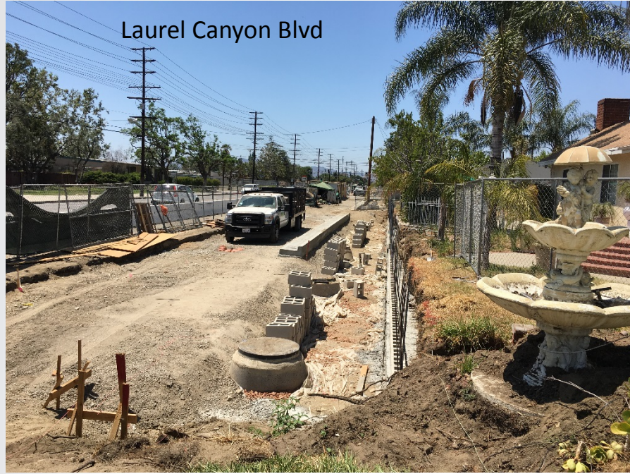
dry wells under construction
