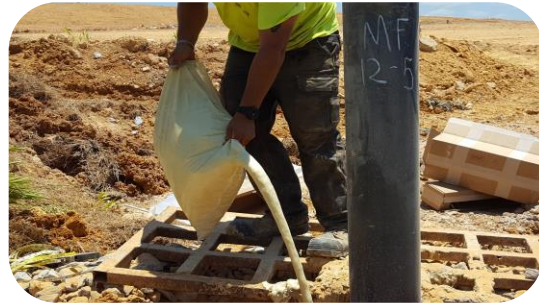
Pouring foam around a well casing
