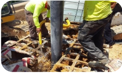
Hydrating bentonite to seal a well
