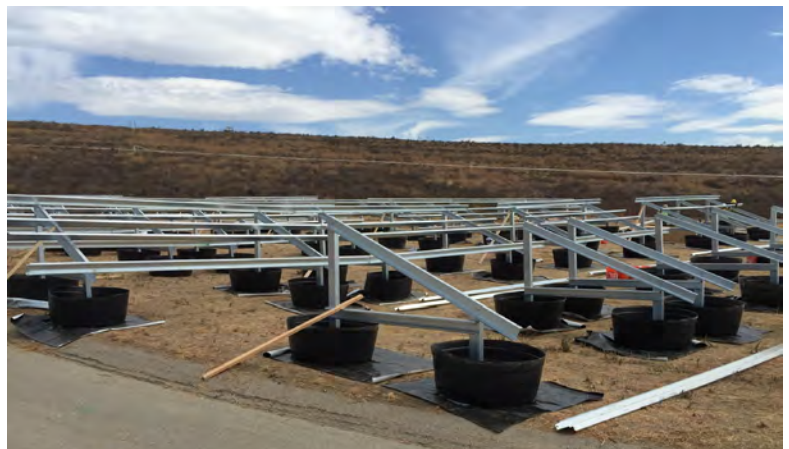
Racking and tubs installed on the Milliken Landfill site.
