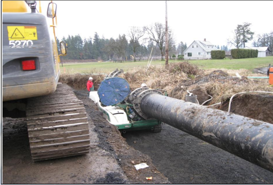
Installation of Irrigation Water Distribution Pipeline (Source: Farmers Irrigation District).
