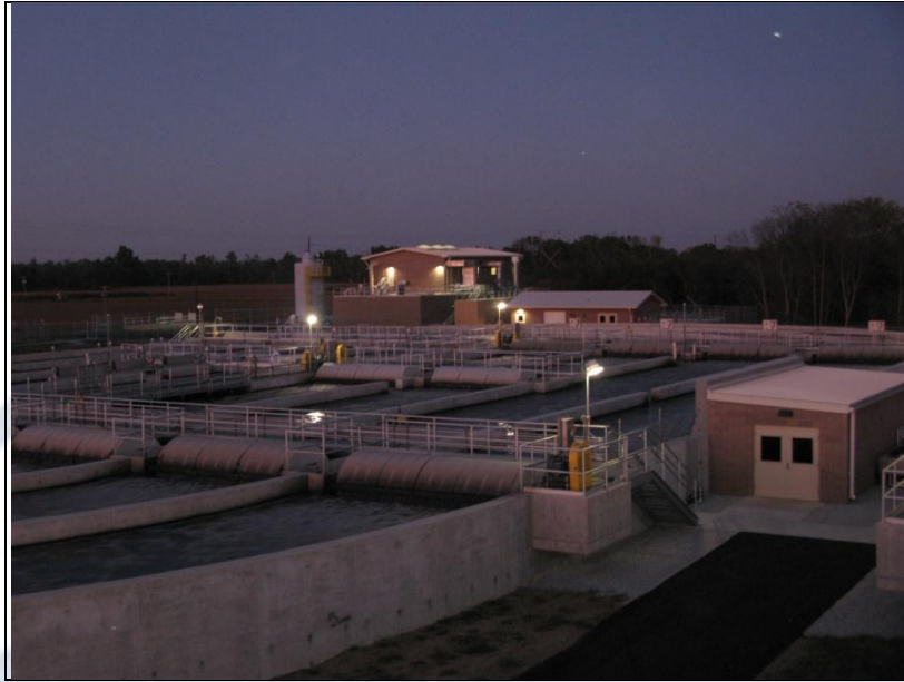
Oxidation ditch process at the Facility (Source: City of Columbus).
