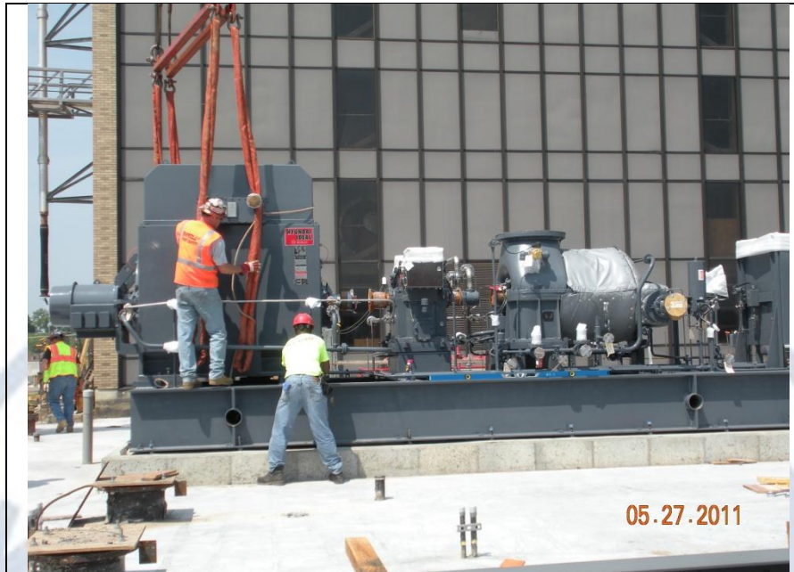
Installation of 1.75 MW Turbine Generator.
