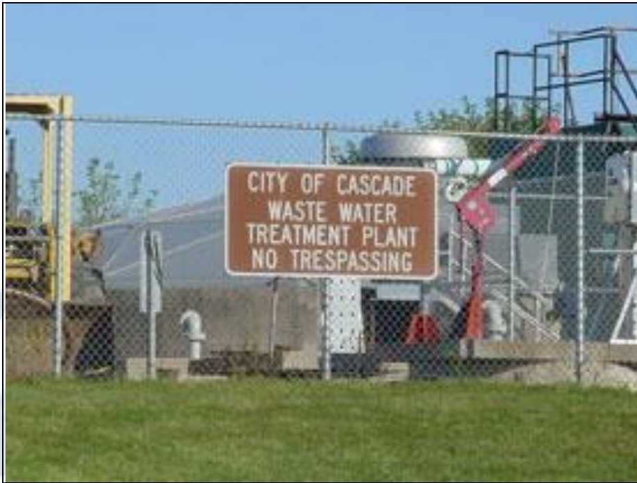
City of Cascade Wastewater Treatment Plant (Source: City of Cascade).
