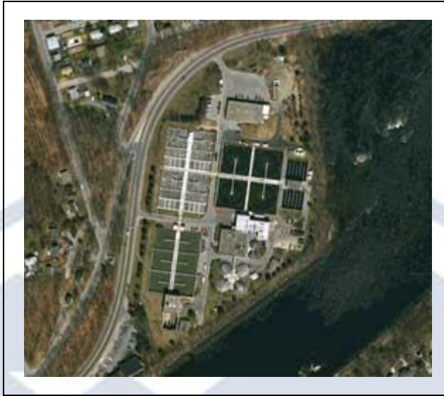
Lowell Regional Wastewater Plant (Source: http://www.mass.gov/dep/water/wastewater/empilot.htm ).
