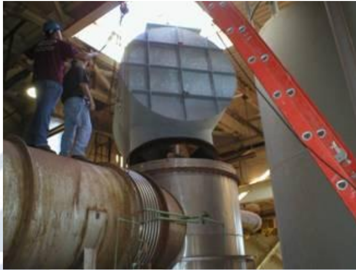
Installation of New Incinerator (Source: AECOM).
