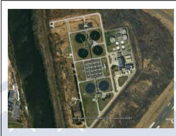
Greater Lawrence Sanitary District Wastewater Treatment Facility (Source: http://www.mass.gov/dep/water/wastewater/empilot.htm ).
