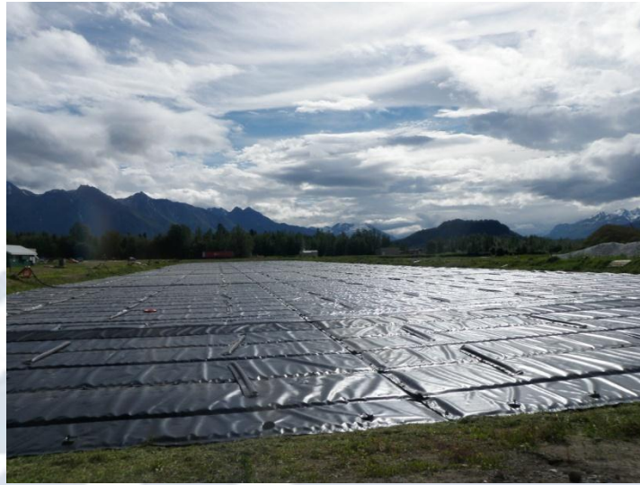
City of Palmer Wastewater Treatment Plant Lagoon (Source: City of Palmer).
