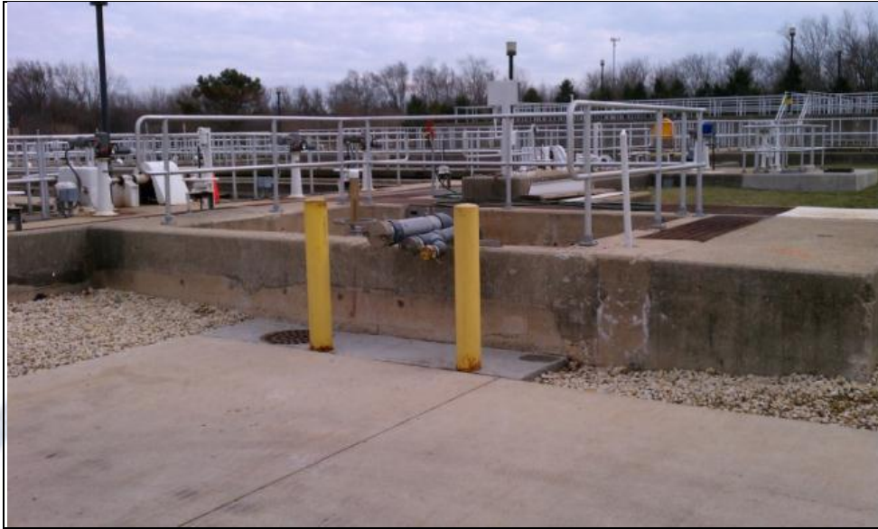
Downers Grove Wastewater Treatment Center Grease Receiving Station (Source: Downers Grove Sanitary District).
