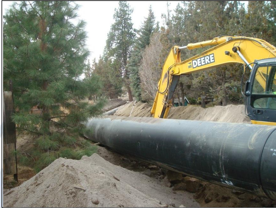
Irrigation Water Pipeline Installation (Source: Swalley Irrigation District).
