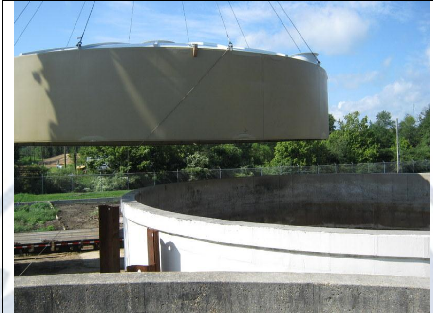
Installation of Digester Cover (Source: City of Moultrie).
