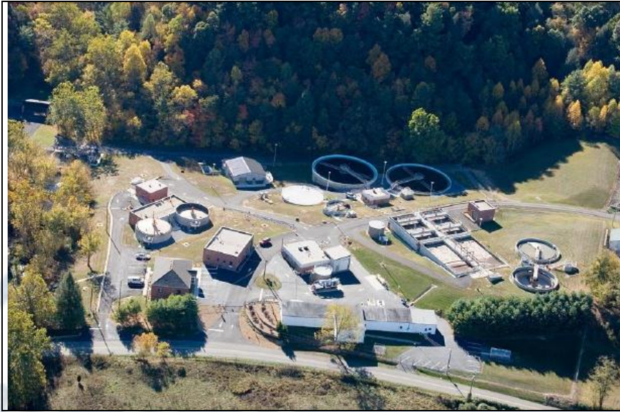
Wolf Creek Water Reclamation Facility (Source: Town of Abingdon).
