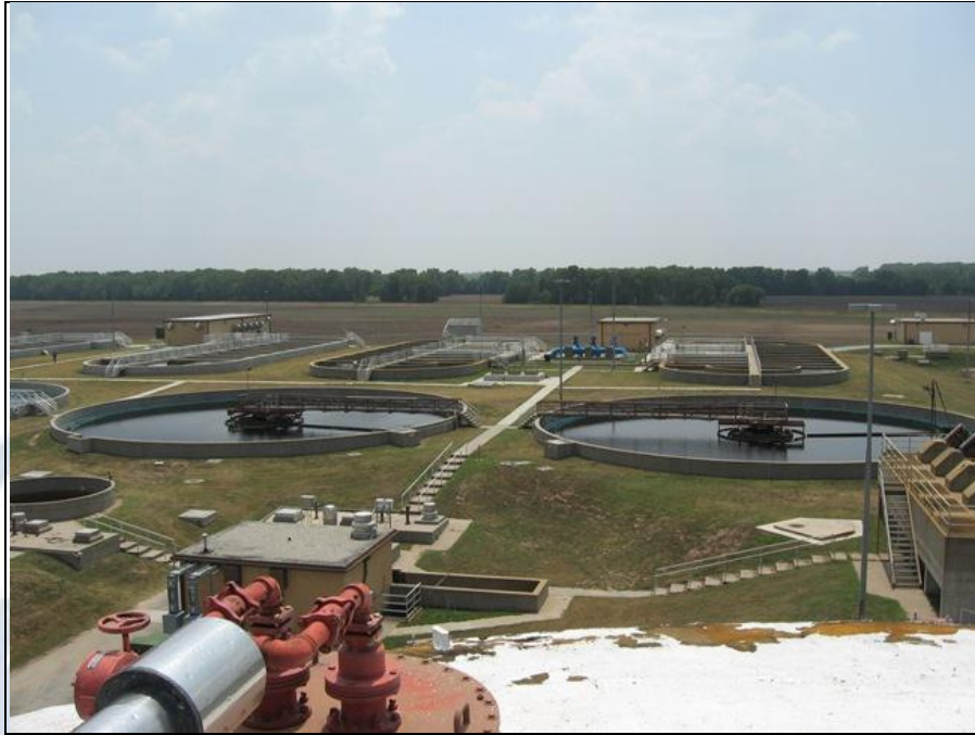
Hutchinson Wastewater Treatment Facility (Source: http://www.hutchgov.com/departments/division.php?fDD=23-112 ).
