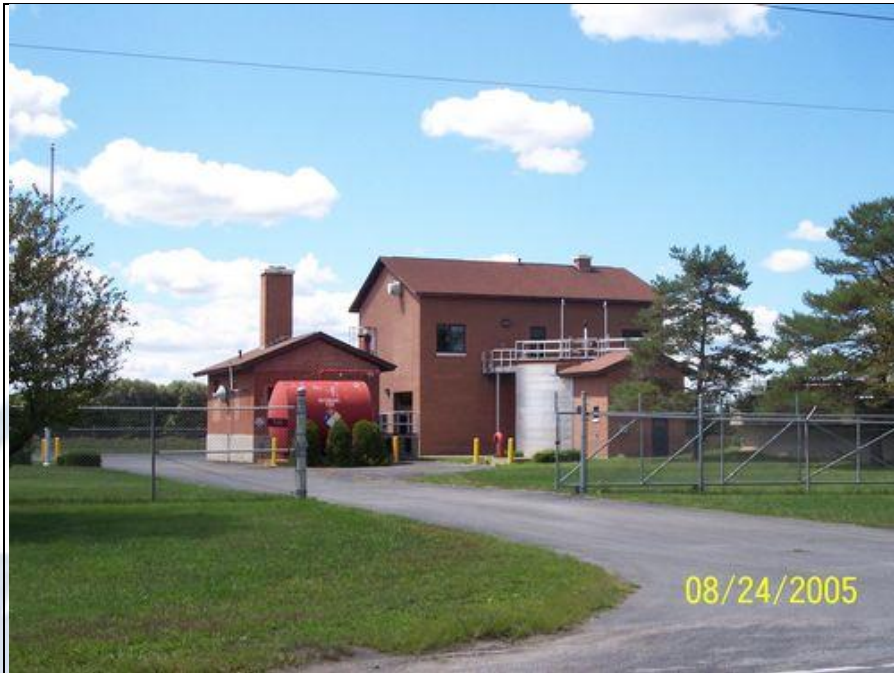
Canastota Wastewater Treatment Plant (Source: http://www.canastota.com/organization.asp?key=45 ).
