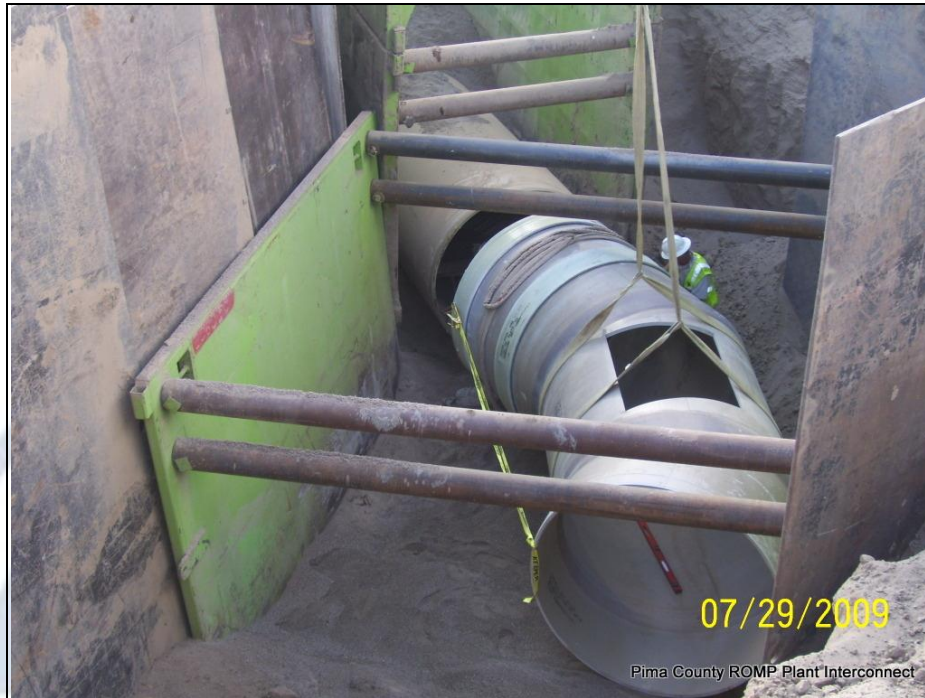
Installation of the Plant Interconnect Pipeline (Source: Pima County).
