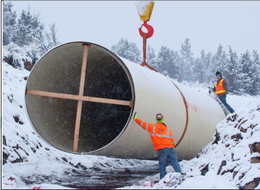
Installation of Irrigation Water Distribution Pipeline (Source: Central Oregon Irrigation District).
