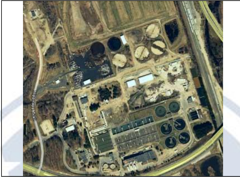
Upper Blackstone Wastewater Treatment Facility (Source: http://www.mass.gov/dep/water/wastewater/empilot.htm ).
