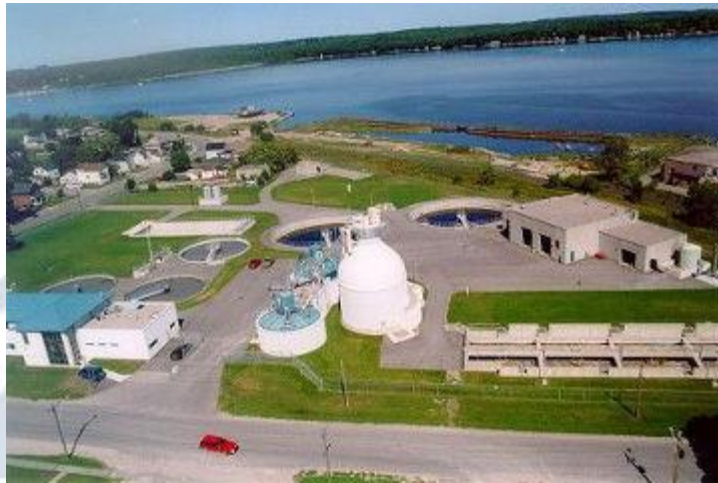
Midland Gas to Energy Project (Source: http://www.waste-management-world.com/etc/medialib/new-lib/wmw/online-articles/2011/01.Par.10696.Image.gif?direct=1 ).
