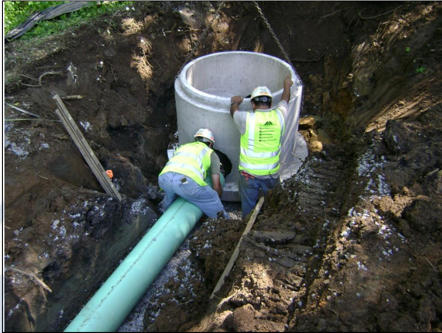
Installation of Gravity Sewer and Manhole (Source: Corporation of Shepherdstown).
