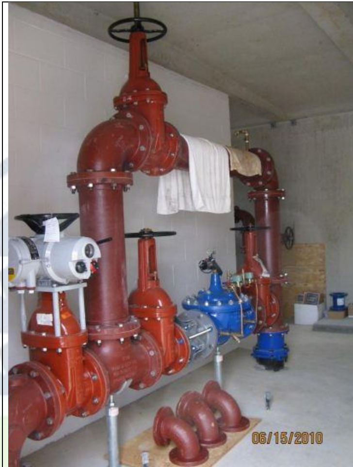
Recycled Water Distribution Manifold (Source: New Kent County).
