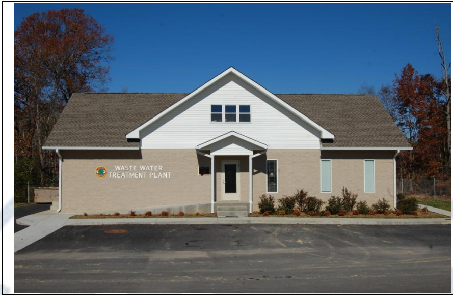
Summerville Wastewater Treatment Plant (Source: http://www.summervillega.org/departments/waste-water-treatment-plant/ ).
