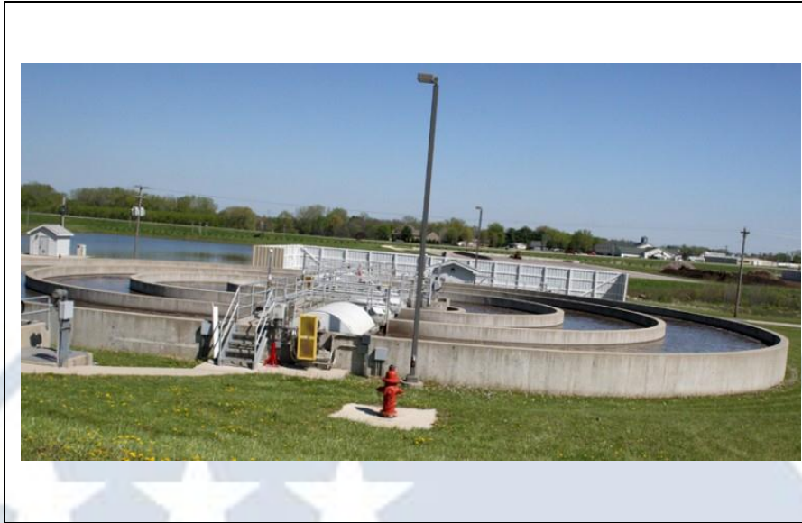
Dyersville Sewage Treatment Plant Orbital Oxidation Ditch (Source: http://www.dyersvillecommercial.com/news/top_news/wastewater-again-hot-topic-for-council/article_79f99c24-8955-11e1-ad1b-0019bb30f31a.html?mode=image&photo=0 ).
