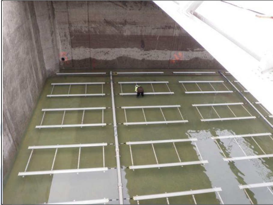
Installation of Diffusers (Source: City of Arlington).
