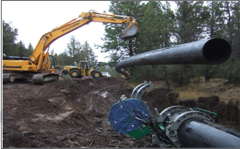
Installation of Irrigation Water Distribution Pipeline (Source: Three Sisters Irrigation District).
