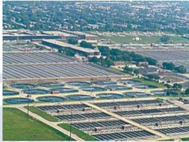
Stickney Water Reclamation Plant (Source: http://www.waterworld.com/articles/wum/articles/print/volume-2/issue-3/Departments/briefs.html ).
