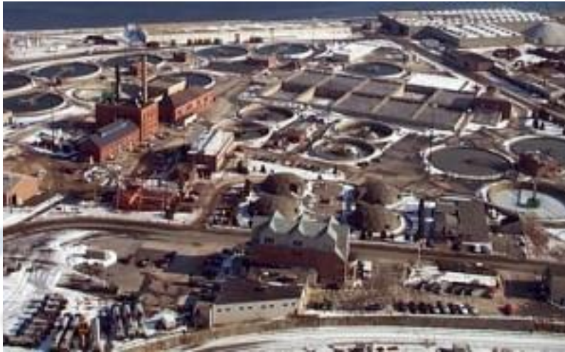
Field's Point Wastewater Treatment Facility (Source: http://www.waterandwastewater.com/plant_directory/Detailed/1005.html ).
