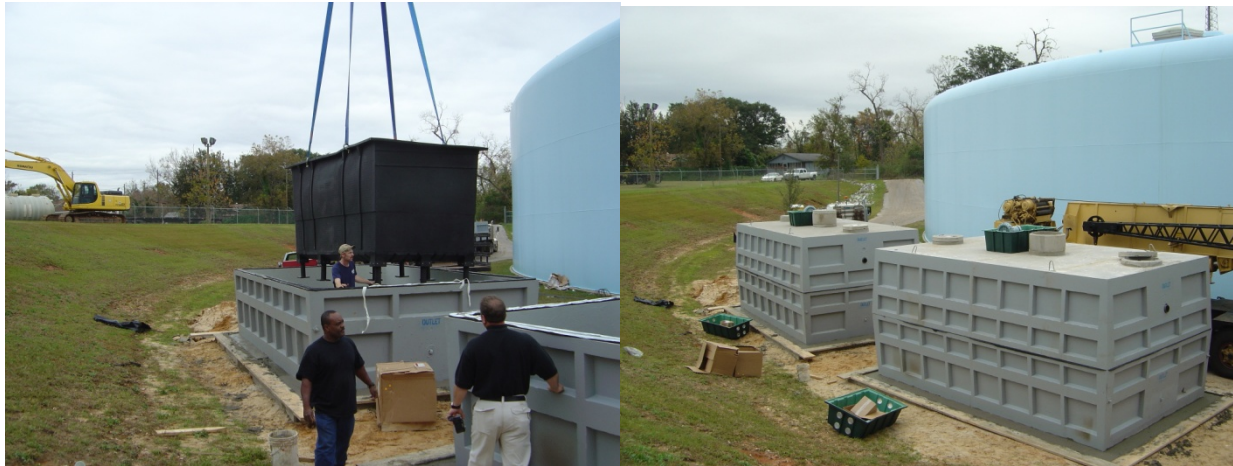
Temporary Community FAST® System in Louisiana, USA
