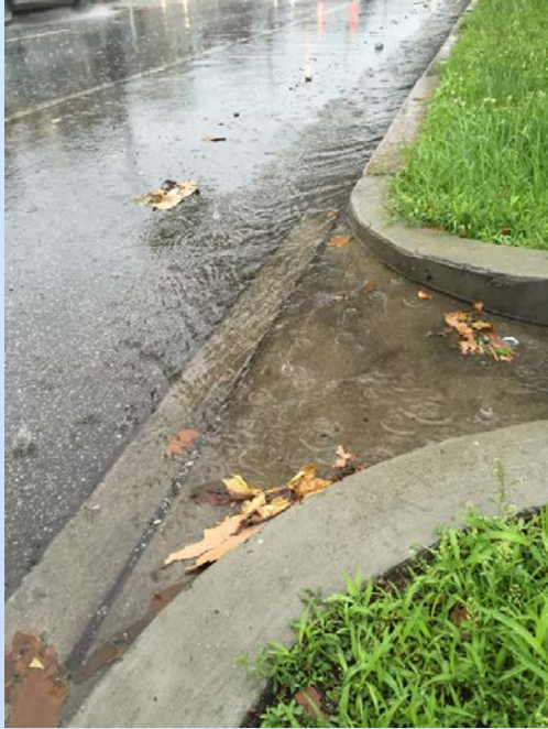
Surface flow bypassing trench drain
